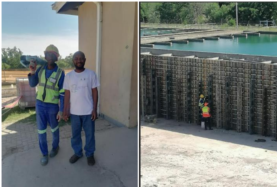
Fig 7. Monitoring of ongoing refurbishment works at the Masselspot drinking water treatment plant in Bloemfontein. The plant supply drinking water to Bloemfontein and was severely sampled, monitored for the emerging contamination project. The project facilitated the prioritisation of the ongoing refurbishment.
